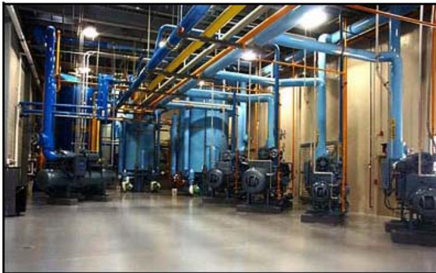
**Fig.3.2.** Ammonia based refrigeration plant for a large cold storage
